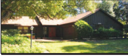
CLASSIC, AFFORDABLE POOL HOME!! Incredible buy, 3BR., 2BA. home, new roof, fresh exterior painting, formal living rm. plus fam. rm. with fireplace, quality block constr., N. DeLand close to major shopping. $185,000. #V4617274
